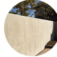
Retaining wall paint
